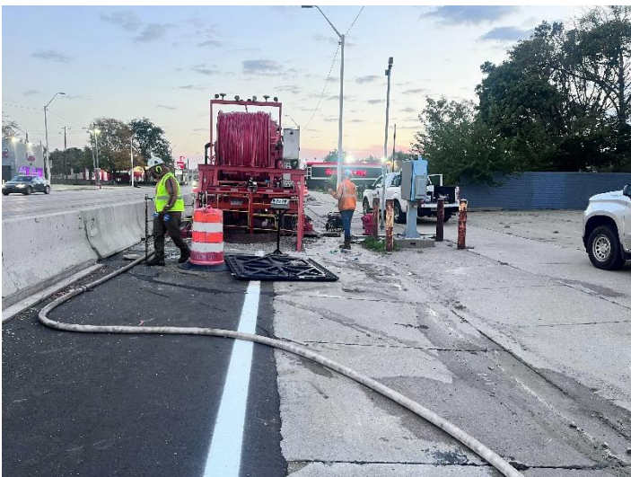
Sewer jetting through MH-102
