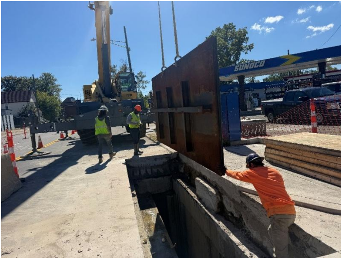
Stop log installation at VR-15
