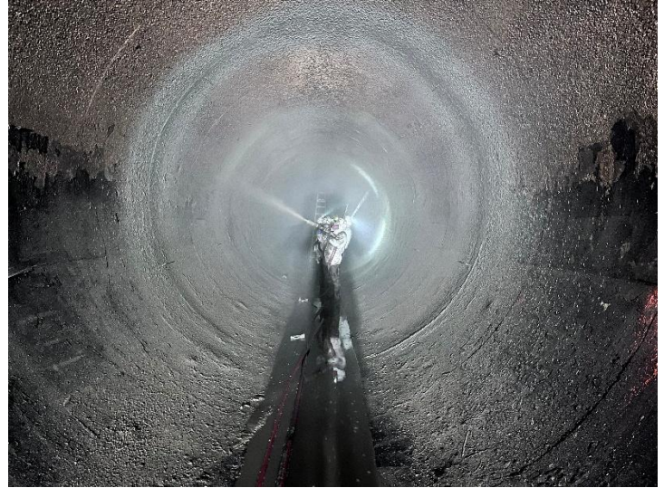
Spray-Lining in PCI-19
