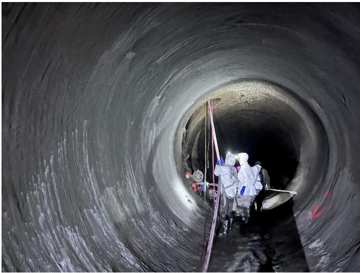
Set-up for Geokrete Lining in PCI-19
