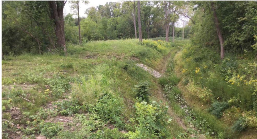
After Drain Maintenance
