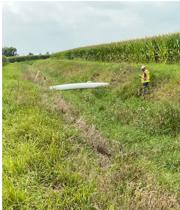
Gas main through county drain
